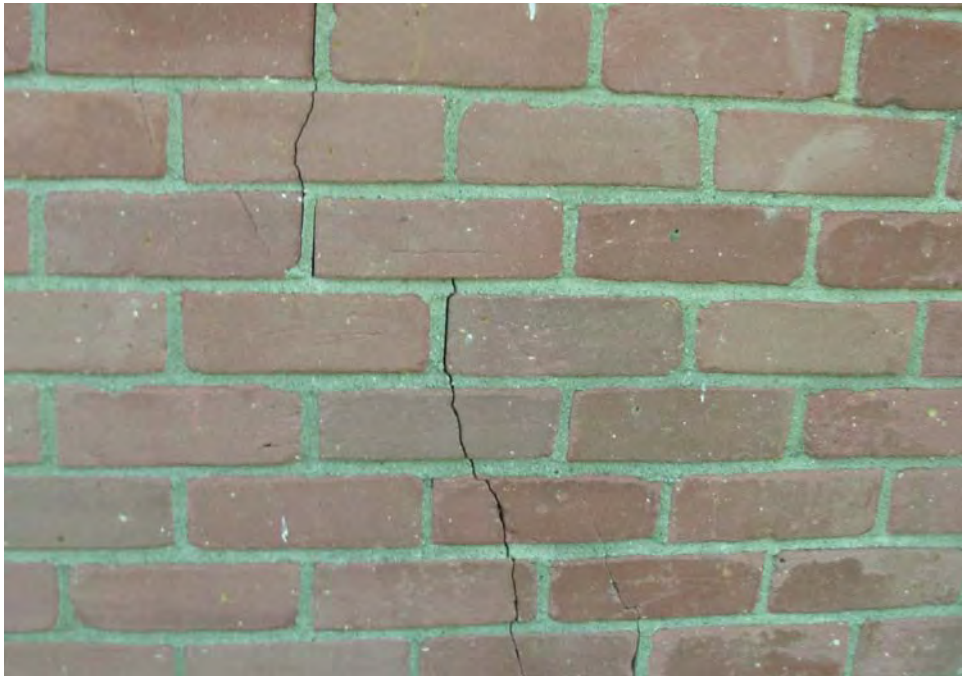
7. Spot brick masonry cracking
