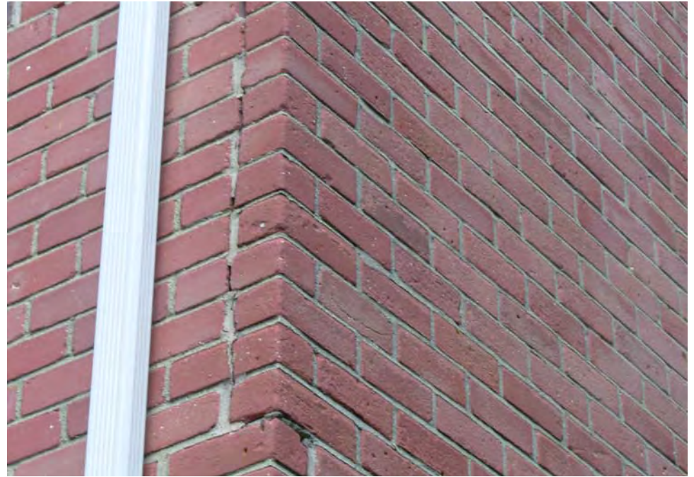
6. Spot mortar deterioration and brick spalling
