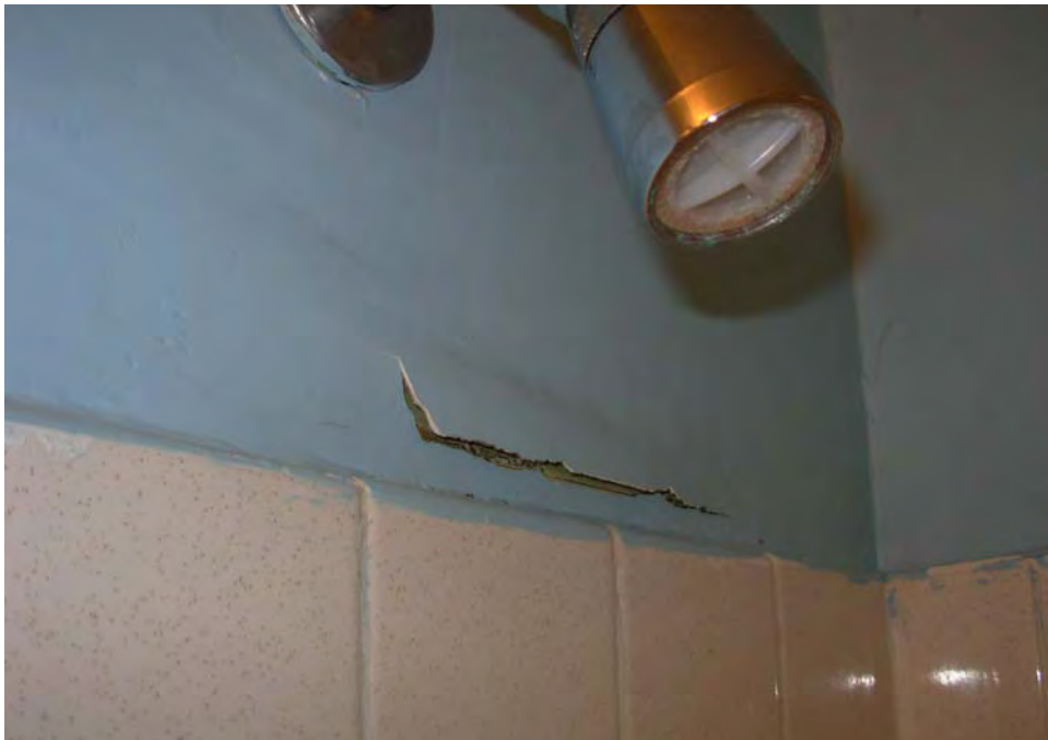
17. Spot wall and tub surround deterioration in unit baths
