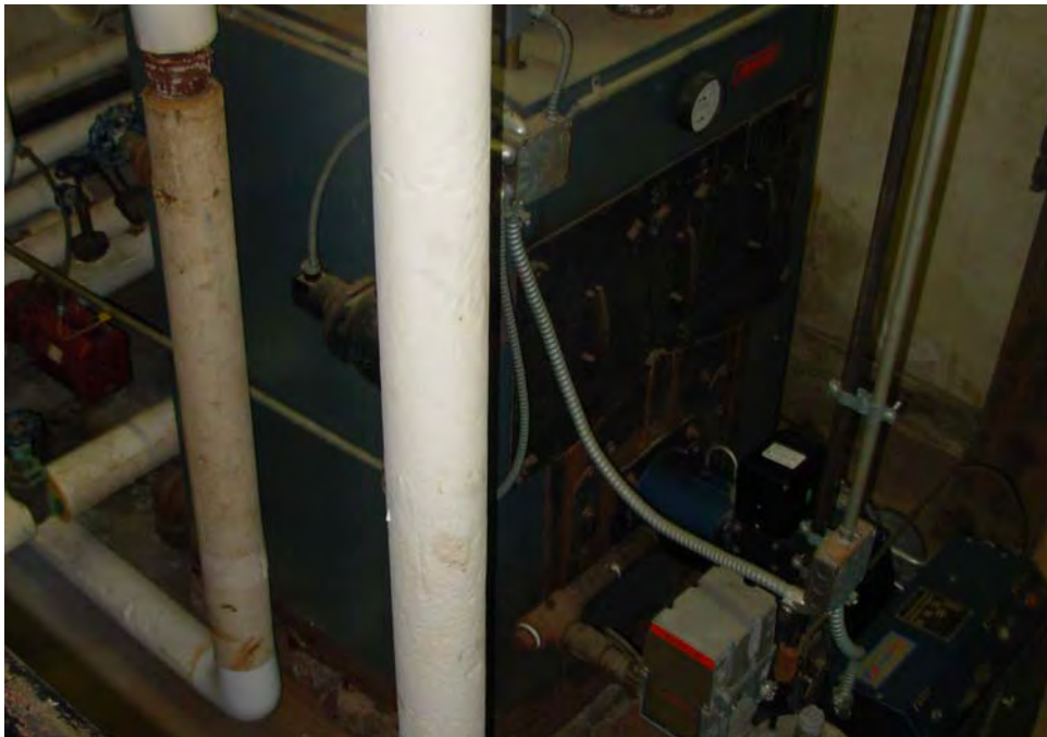
13. Typical heating boiler assembly
