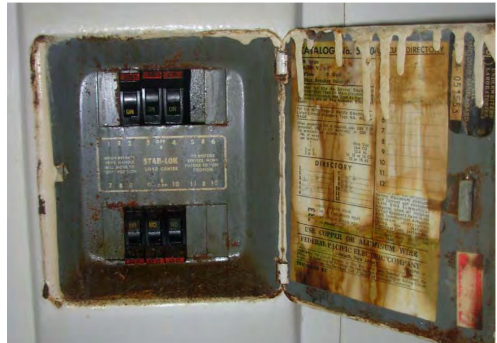
20. FPE Stablok circuit breaker panels, to replace
