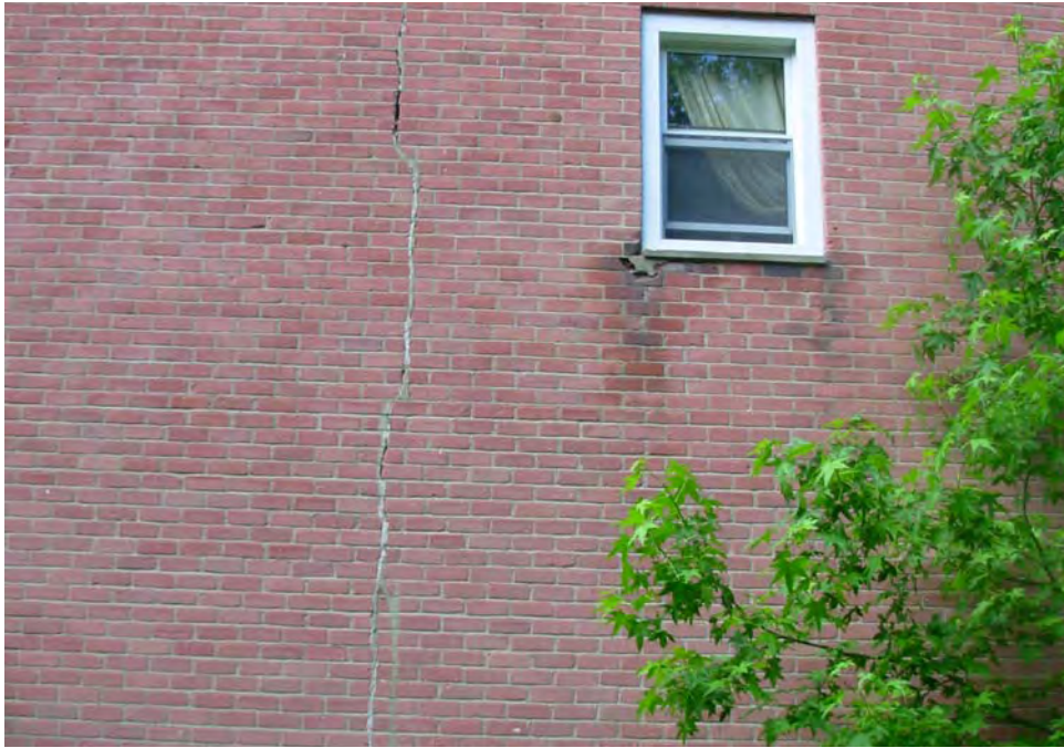
5. Vertical cracking at gable end wall of one building
